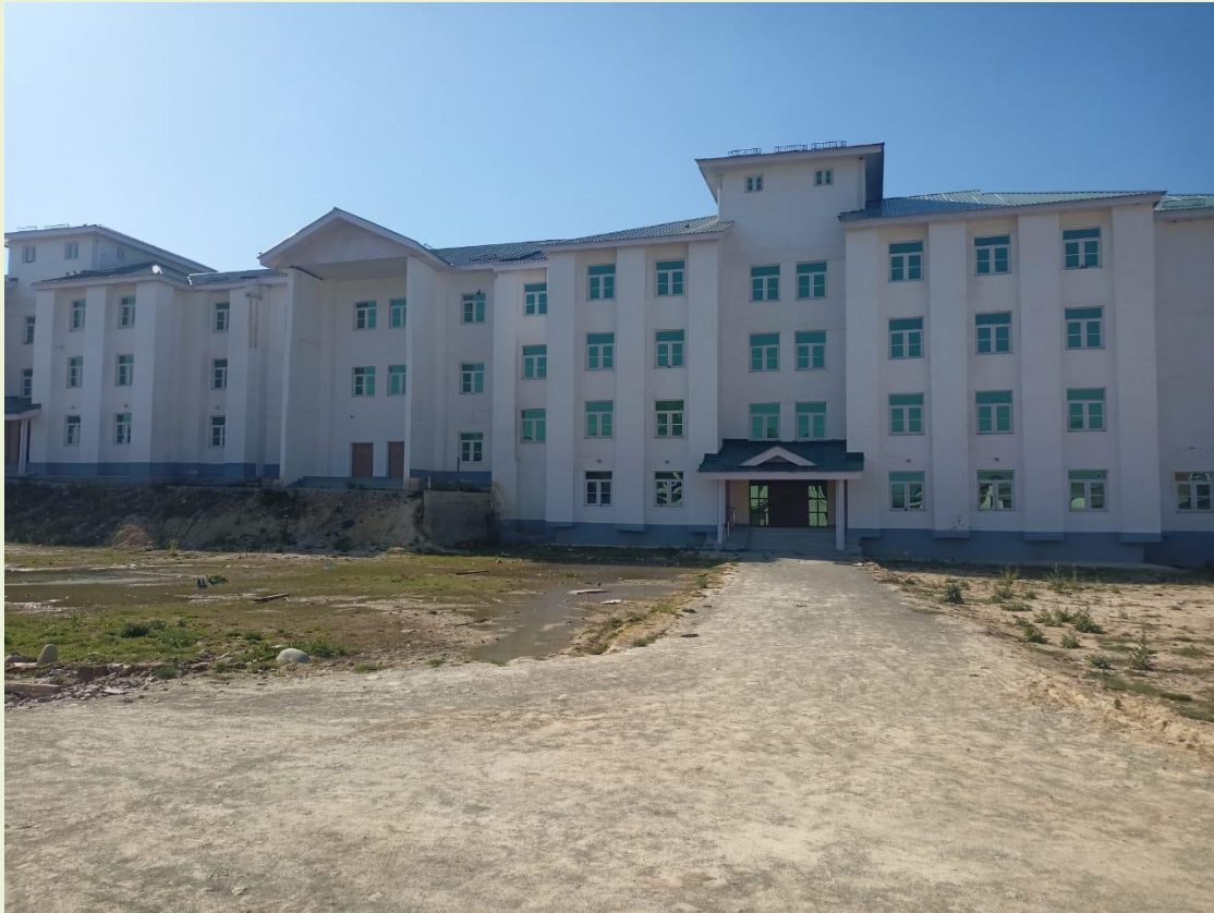
New Hostel Building with capacity of 180 students (boys and girls), with dinning facility also
