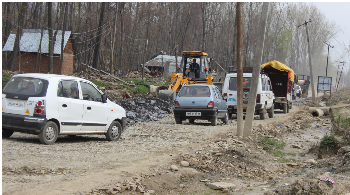
Vehicles plying on dilapidated Srinagar-Jammu national highway. AABID BHAT/IUST
